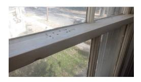
• Attention: The inspector was unable to get some of the older windows open. The windows appeared to be painted shut. Freeing up the windows may be considered in order to provide ventilation for the structure and allow proper egress in case of emergency.
