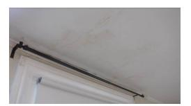
• Action required: There were moisture stains evident on the living room ceiling, kitchen ceiling, and rear lower close ceiling that tested dry at the time of the inspection. The exact origins could not be confirmed. A further evaluation by a qualified contractor is recommended.
