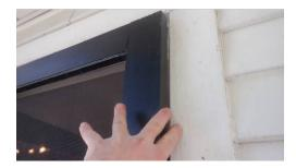
• Attention: There was a key lock installed for the rear exterior door. This is not a recommended arrangement due to the difficulty of egress in the event of an emergency. Installing a standard dead bolt is recommended. Contact a qualified contractor to make a further evaluation and the necessary modifications.
