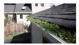
• Action required: In order to improve the site drainage, it is recommended to discharge the rain water 4'-6' away from the house wherever possible. Down spouts that empty along the foundation wall is the most common cause of deterioration to foundation systems.
