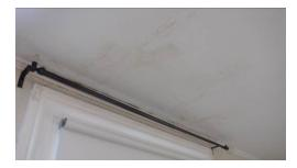
• Action required: There were moisture stains evident on the living room ceiling, kitchen ceiling, and rear lower close ceiling that tested dry at the time of the inspection. The exact origins could not be confirmed. A further evaluation by a qualified contractor is recommended.
