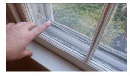
• Action required: A random test of the windows was done to see if they could be latched/locked and opened/closed. The test revealed that the majority of the older windows in the structure have broken balances. The windows will not stay in the desired position without a prop. Repairs are necessary as windows with broken balances are a potential safety hazard and eliminate an egress in the event of a fire.
