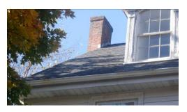
• Multiple roofing layers were noted. Only up to 2 layers of roofing material are allowing as per local ordinances, as well as to help prevent damage to the roof sub-structure from excessive weight. At time of re-surfacing, all roofing layers will need to be removed.
